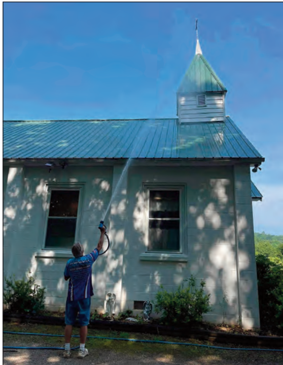
Bill Hutson pressure washes a metal roof on a church.
