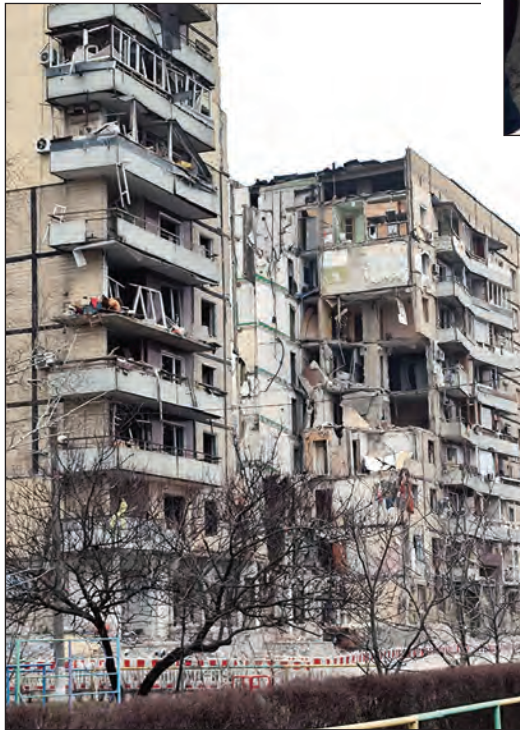
A common sight that missionary Loren Kennedy experiences during his trips to Ukraine are those of bombed-out apartment buildings.
