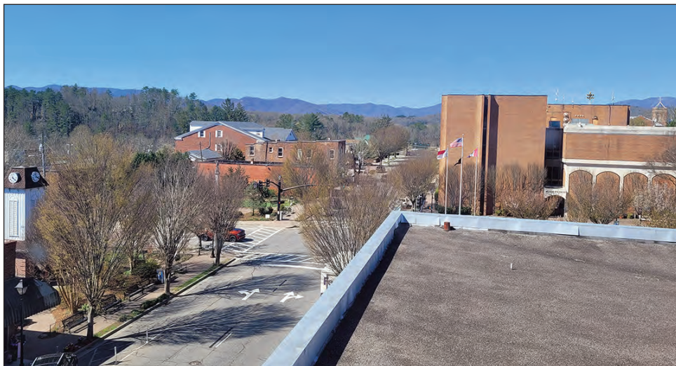
A rooftop restaurant, with views of surrounding mountains, is envisioned for the boutique hotel project.
