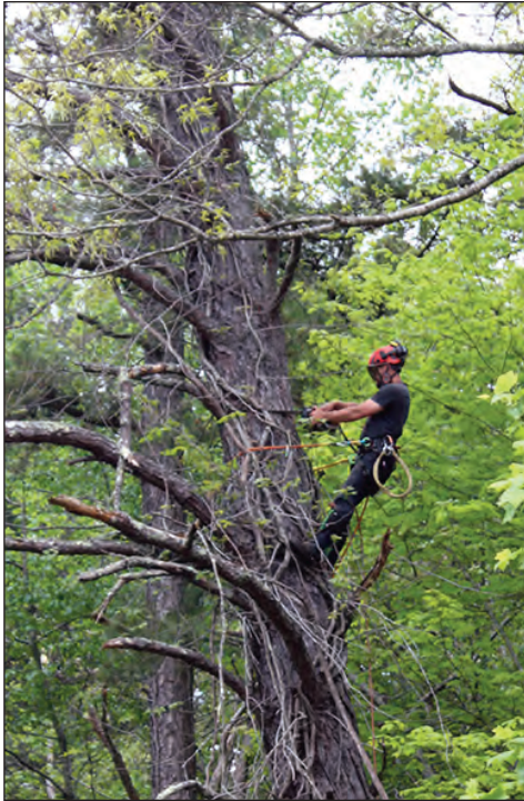
Recently the Lee Talley Tree Company took down a yellow pine tree that was threatening a nearby structure. Tree climber Brandon Elliott wielded the saw, first cutting the top of the tree, as crane operator Luke Cook guided it and two other sections to the ground where it was cut into 12-foot logs by Dustin Daves and Lee Talley. The process took about two hours. Photos by Betsey Gooder
