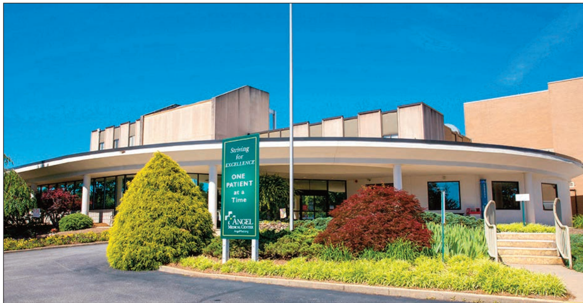
Angel Medical Center is slated to be replaced with a new facility just off the 441 bypass. HCA spokesperson said construction was slated to begin in late 2020. Photo by Vickie Carpenter
