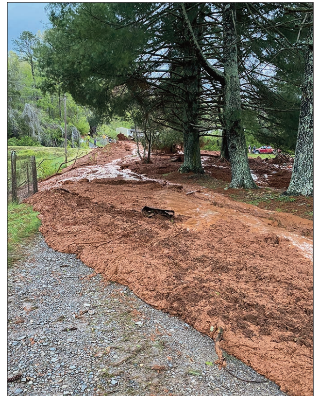
The Pressley Road mudslide continued down the mountain but no other structures were affected.
