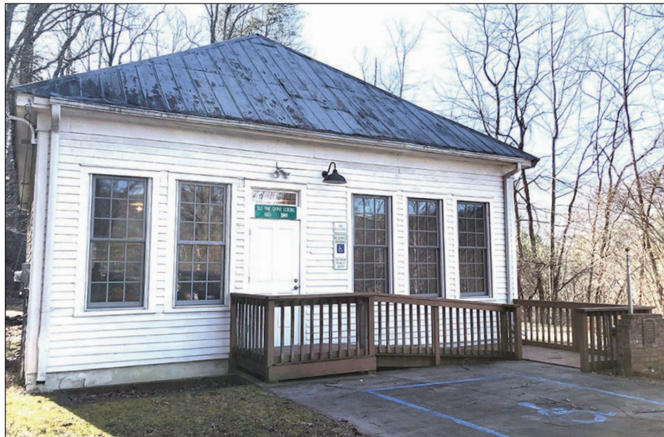
Pine Grove School was restored in 2006 and is now used as a community building.
