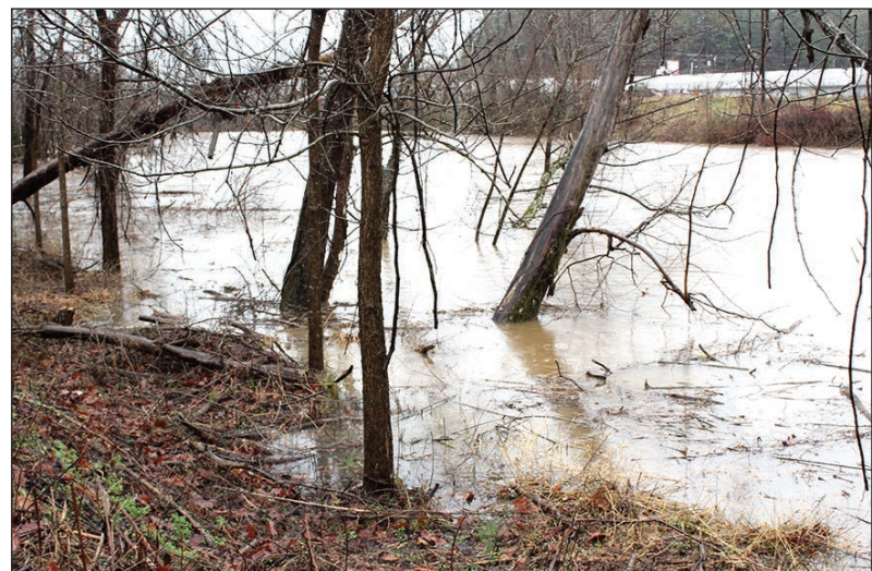
According to Mike Cope with the county maintenance department, the major damage caused by flooding along the Greenway is to the eroding river banks.
