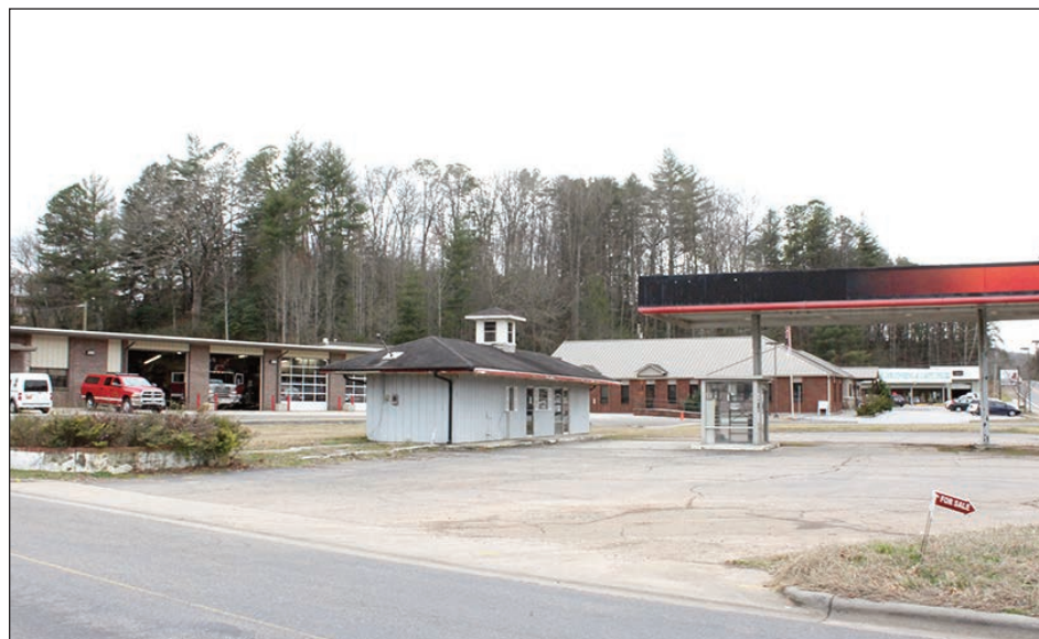
The Town of Franklin is poised to close on the old Texaco property directly in front of the Franklin Fire Department at a cost of $180,000. According to Town Manager Summer Woodard, the property will be useful for the town for sidewalk and water/sewer line projects as well as to enhance the properties surrounding the parcel. Photos by Vickie Carpenter
