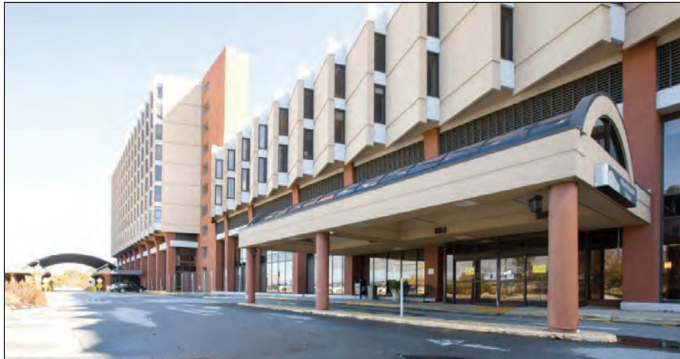
The St. Joseph's building is one of the older facilities belonging to Mission Health in Asheville. Colby Rabon / Carolina Public Press
