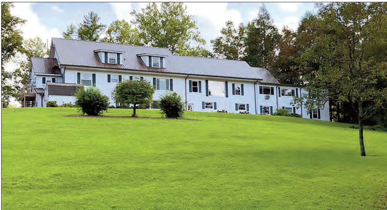
Around 1948, the 13-guest room, 11-bathroom inn was built as a resort and named Wayah Valley Inn. It is now headquarters for the Christian Training Center. CTCI, just off Wayah Road, overlooks Wayah Bald and the expanse of mountains flanking the fire tower summit.
