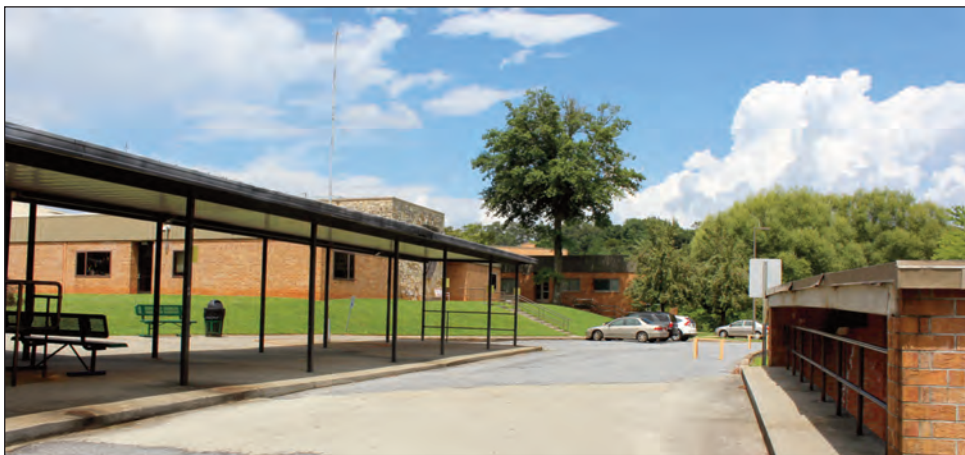
Macon Middle School students can look forward to new floors, brighter lighting systems and new color schemes. Classrooms will be moved around to accommodate projects still underway as the new school year begins Aug. 23. Photo by Vickie Carpenter
