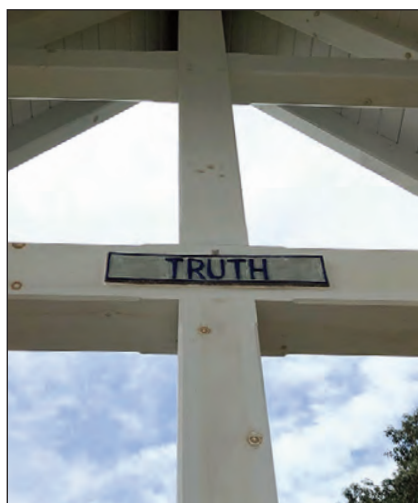
All four sides of The Grove pavilion include handmade plaques by a local potter, and the east and west sides are crosses. The arbor is complemented by a landscaped area with benches.
