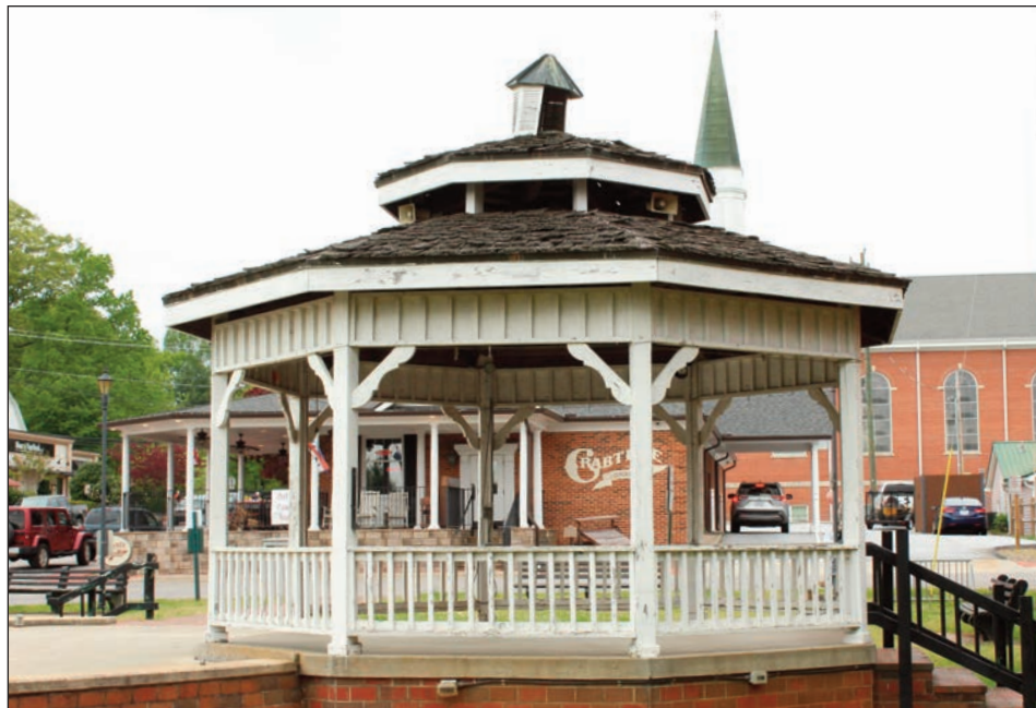
An overhaul for the gazebo on town square in downtown Franklin has been banded about for years. The Town manager is allowing $8,000 in the budget for new cedar shake shingles for the roof and a coat of paint. Photo by Vickie Carpenter
