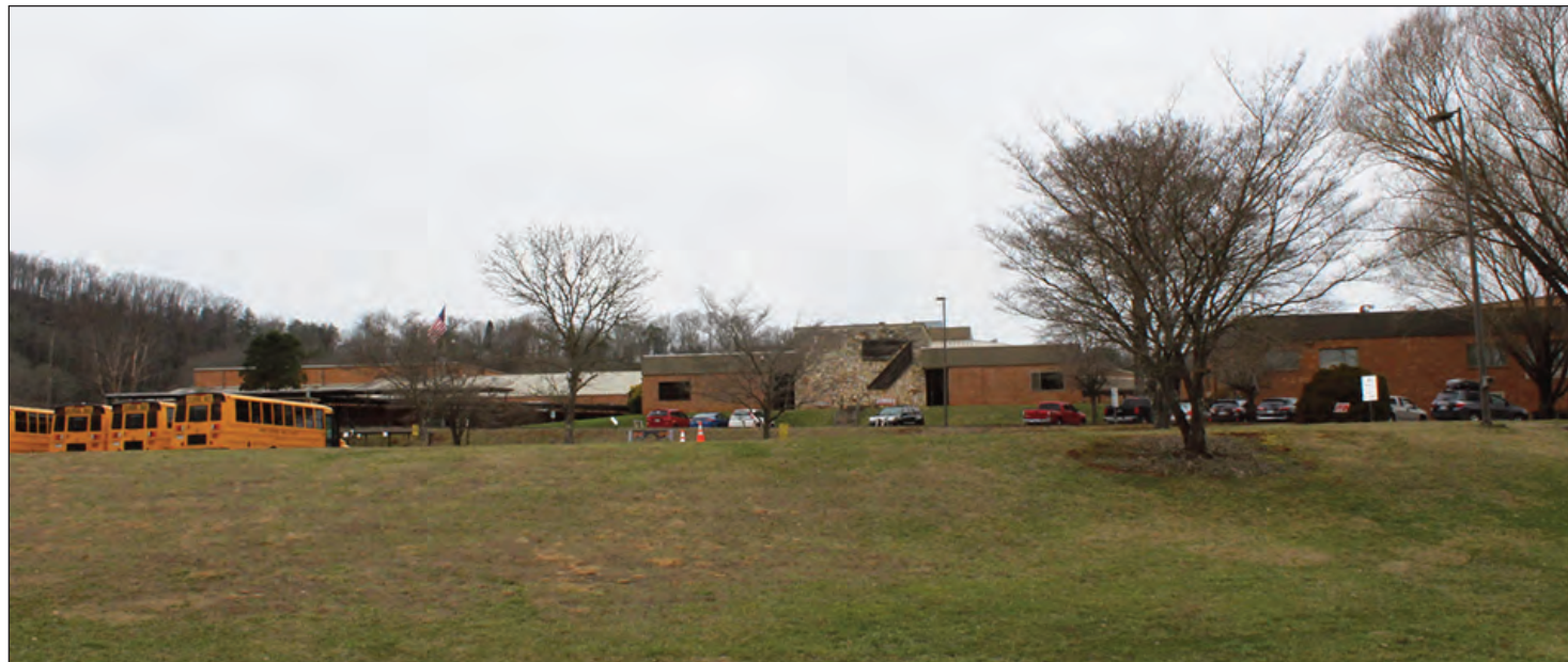
Macon Middle School's much needed renovations have been talked about since 2017. Macon County Commissioners voted Friday to go ahead with the project. Photo by Vickie Carpenter
