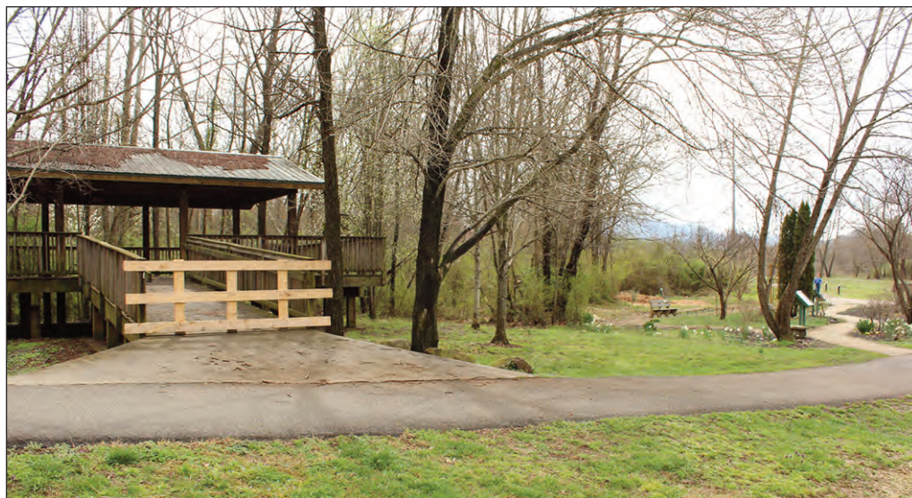
FROGs plans major renovations to the shelter near the Airport Trail portion of the Greenway. Local Rotary clubs will assist with the repairs. Photos by Vickie Carpenter
