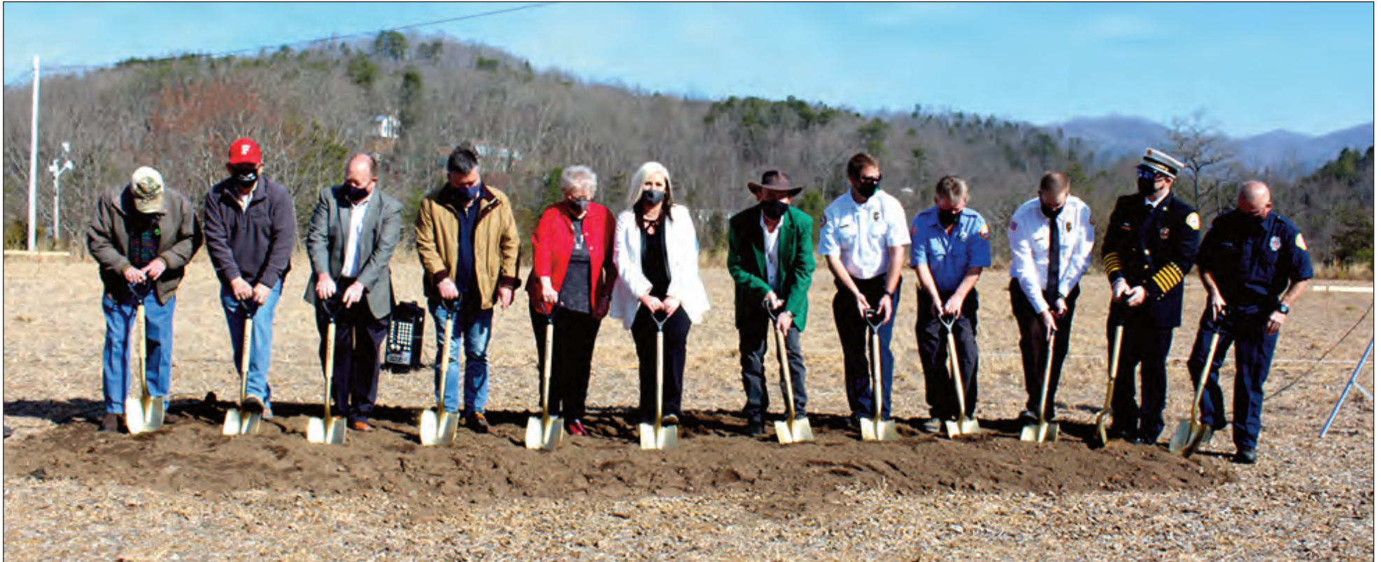
Franklin Fire & Rescue, town officials and others gathered on Wednesday morning to break ground for a new fire substation in NP&L Loop just off Sylva Road. The Town of Franklin purchased the property in August 2019 and hired Ritter Architecture to assist with site drawings, plans and formal bid proposals. The contract was awarded to Western Builders for $399,019 to construct the substation. Construction is set to begin this spring. Pictured (L-R) are Bob Scott, Jack Horton, Joe Collins, Michael Lewis, Dinah Mashburn, Summer Woodard, Tom Ritter, Asst. Chief Ryan Hursey, Max Houston, Captain Justin Setser, Chief Ben Ormond and Chuck Norton. Photo by Vickie Carpenter
