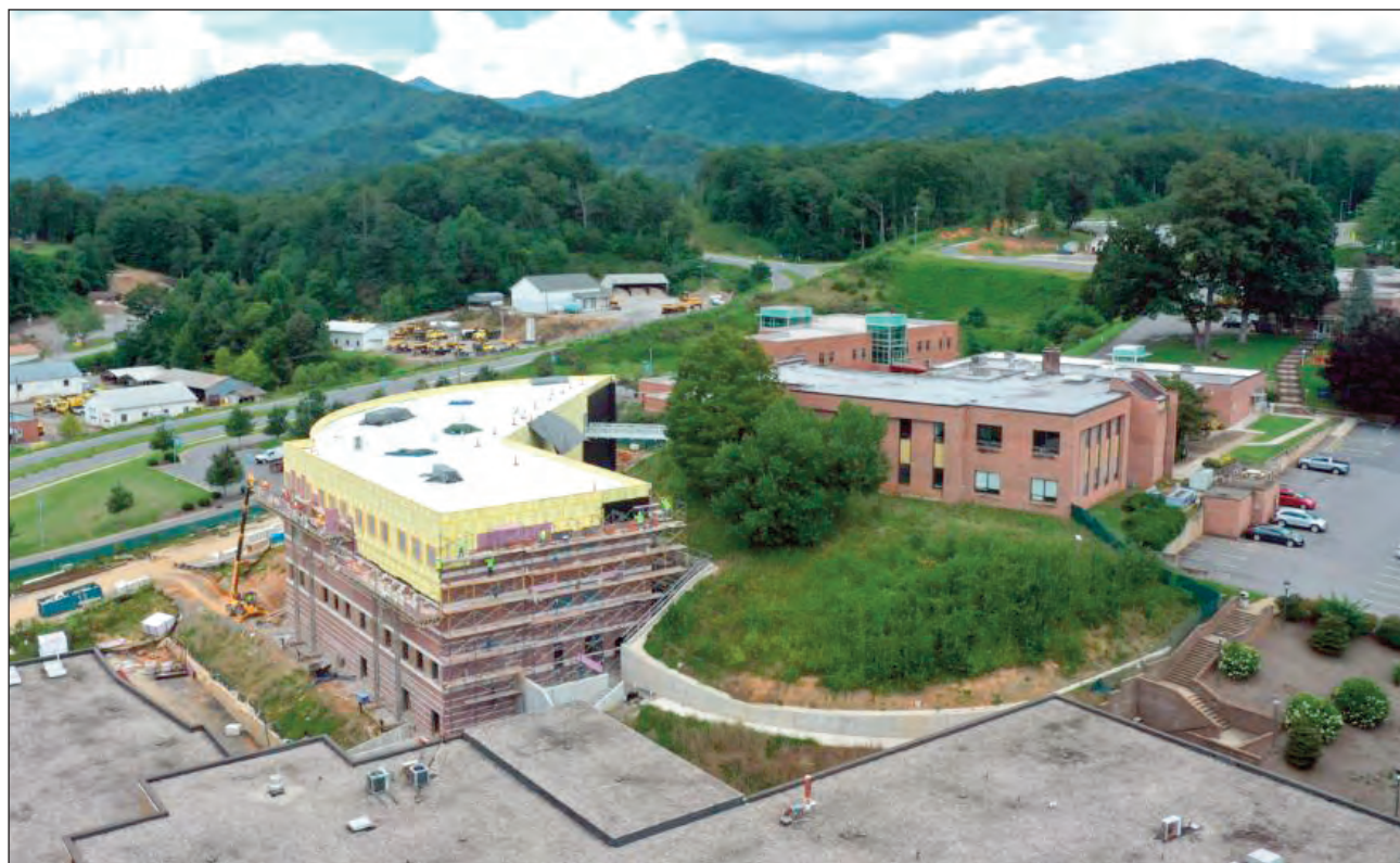
The new health sciences building at Southwestern Community College.
